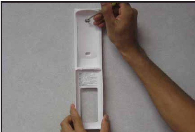
Figure 2. Mounting Remote Control Housing
