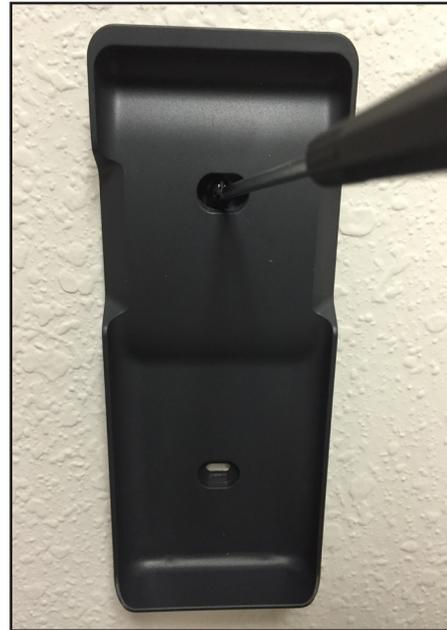
**Figure 6. Install the Wall Mount**
