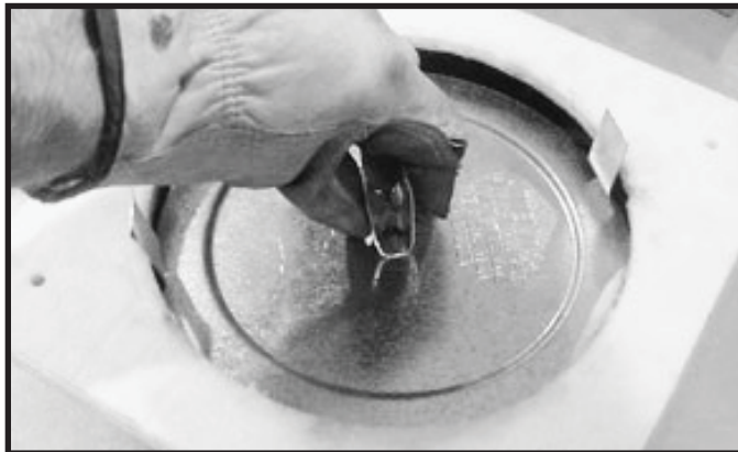
Figure 6.2 Fold the center parts of the retaining band up and use to remove the vent cap.
