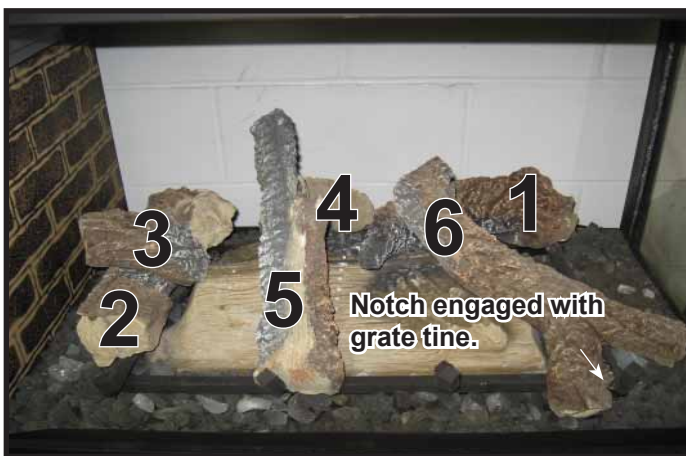
Log Assembly Installed.
