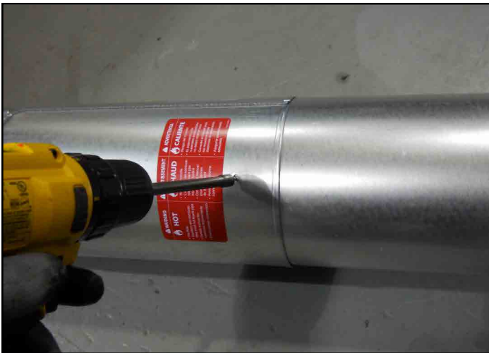
Figure 7.4 Screws into Slip Section
