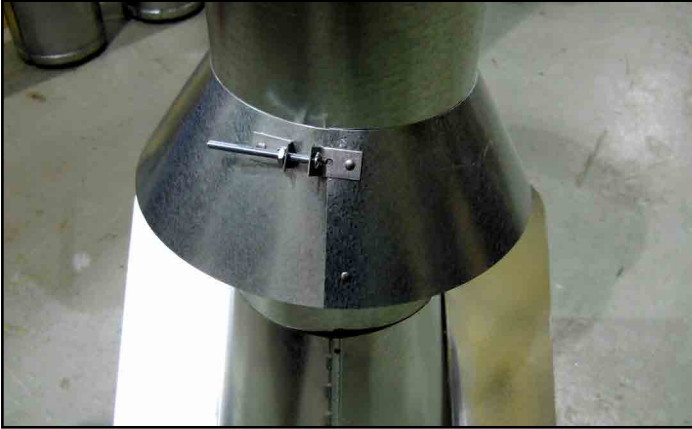
Figure 7.14 insert Bolt into Brackets
