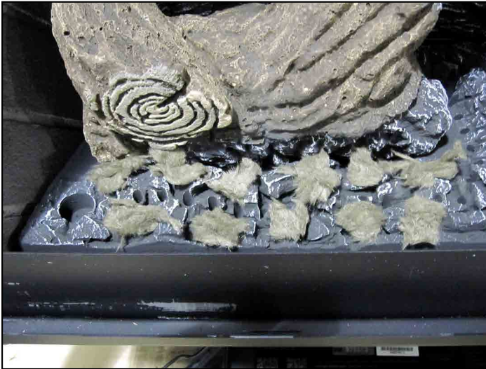
Figure 10.13 Place Mineral Wool
