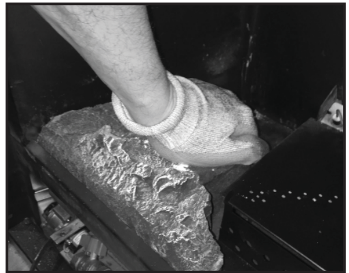
Figure 11.2 Press Left Hearth Firmly Into Place
