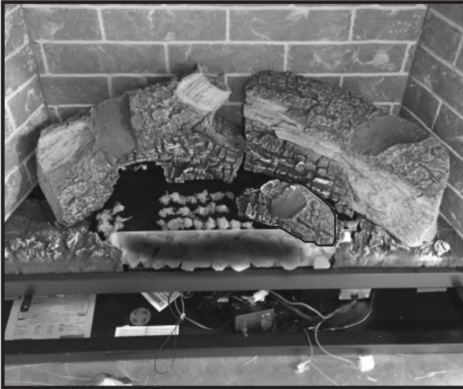
Figure 6. Burner Log Installed
