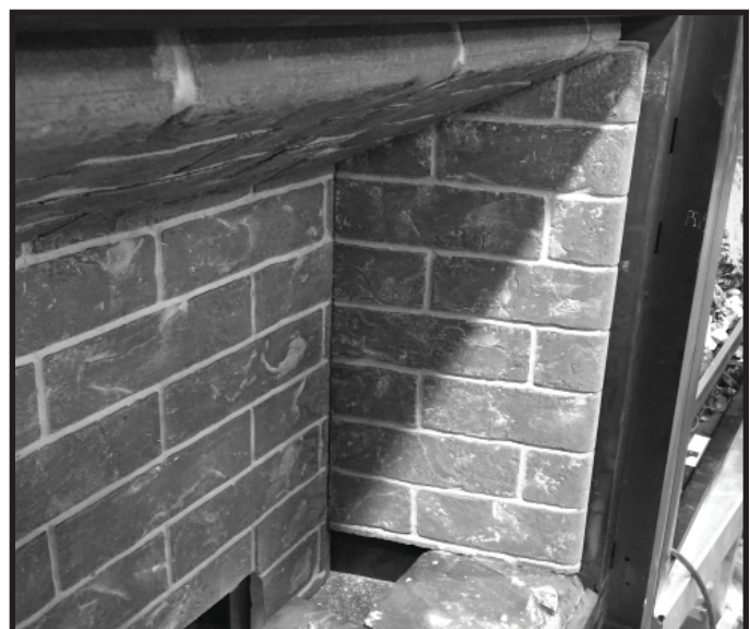
Figure 11.7 Right Refractory Panel Installed
