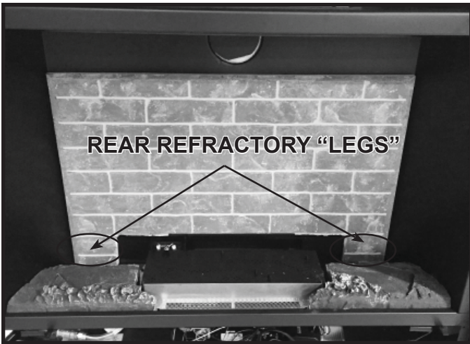
Figure 11.3 Install Rear Refractory Piece
