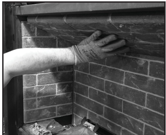
Figure 11.6 Install Right Refractory Panel
