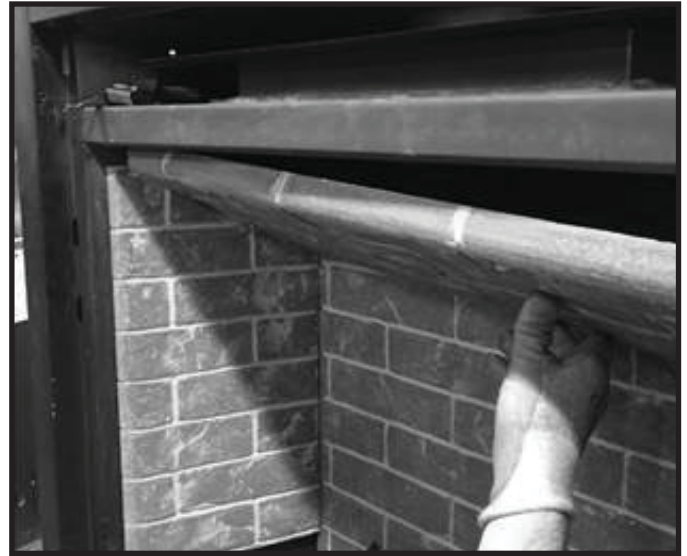
Figure 11.5 Install Top Refractory Panel
