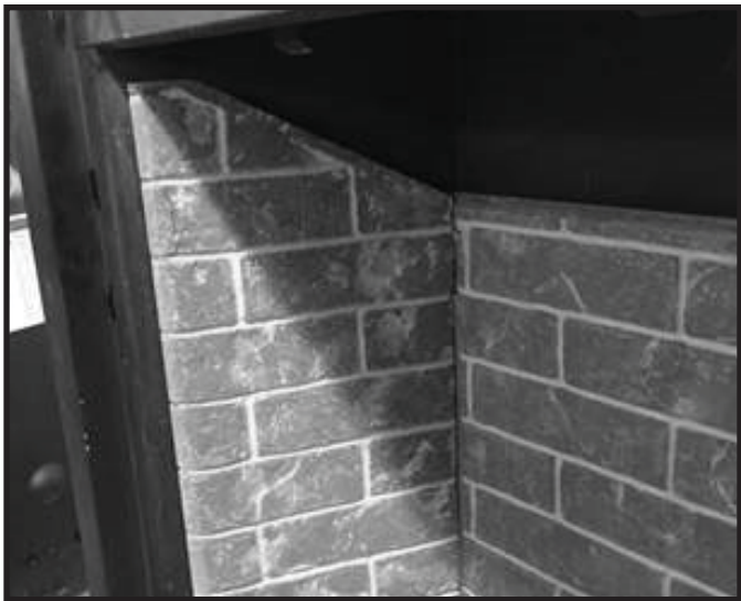
Figure 11.4 Install Left Refractory Panel
