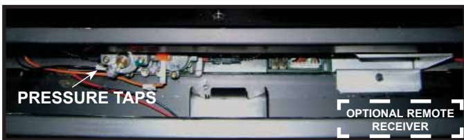
Figure 11.5 Valve Pressure Taps and Remote Receiver Location
