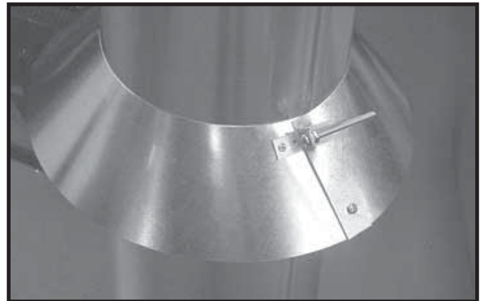
Figure 10.13 Assembling the Storm Collar Around the Pipe
