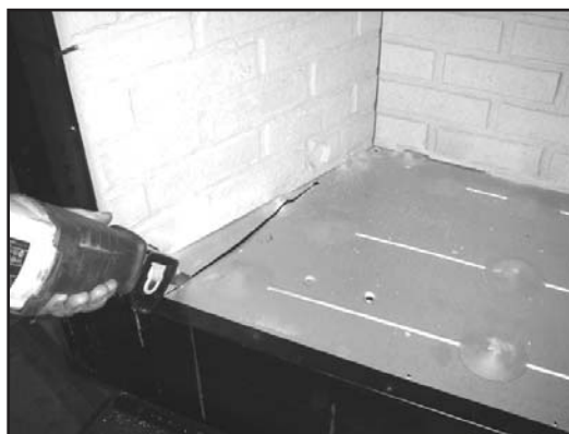
Figure 10.3. Using a sawz-all, cut out the floor.
