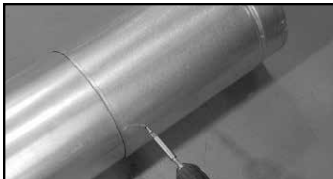
Figure 10.7 Vis de la section coulissante
