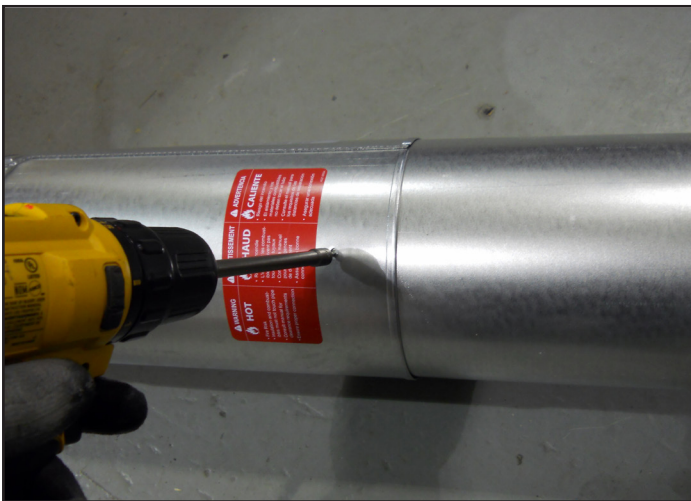
Figure 7.4 Vis de la section coulissante
