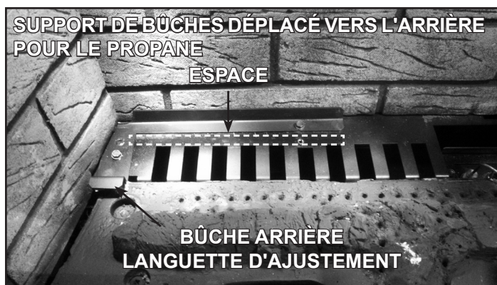
Figure 10.9 Position du support de bûches - propane
