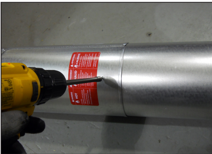
Figure 7.4 Vis de la section coulissante
