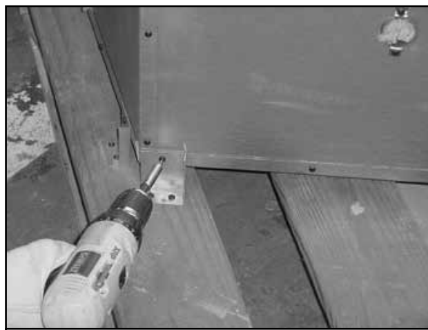
Figure 3.11 Removing Shipping Brackets
