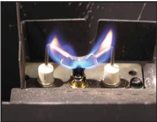
Figure 3.2 IPI Pilot Flame Patterns
