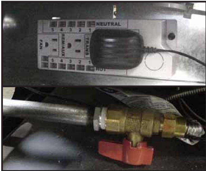
Figure 13.5 Preparation to Install Splatter Guard
