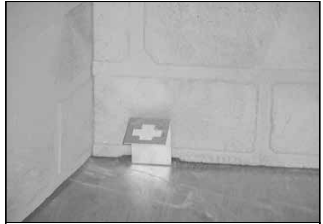
Figure 8.8 Grate Retaining Bracket in Place
