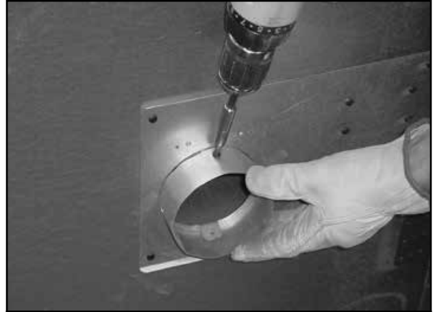
Figure 3.18 Attaching Outside Air Kit Collar
