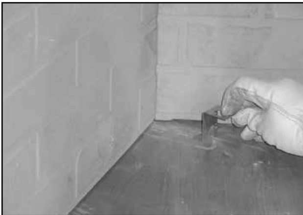
Figure 8.7 Slide Grate Retaining Bracket into Notch
