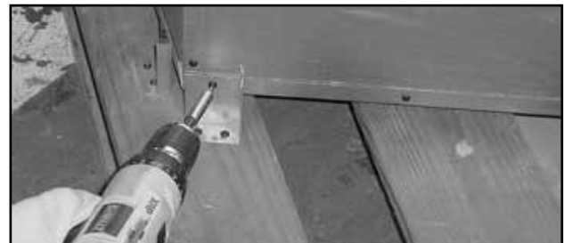
Figure 3.10 Removing Shipping Brackets
