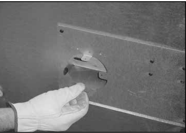
Figure 3.17 Bending Tabs on Outside Air Kit Collar
