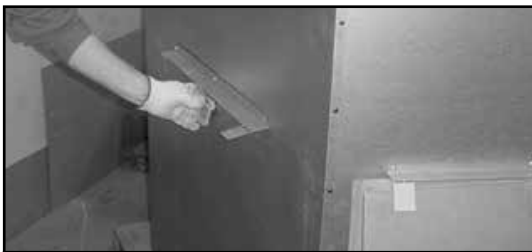
Figure 3.6 Bending Refractory Shipping Tabs Back Down
