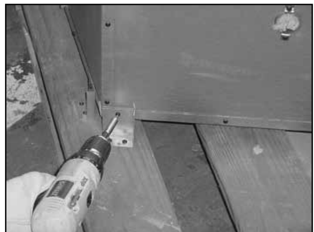
Figure 3.11 Removing Shipping Brackets
