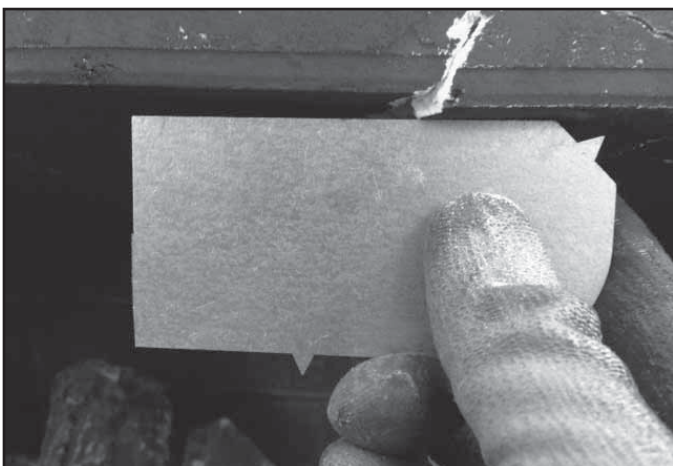
Figure 4.6. Surface plane of firebox is comprised and should be replaced.
