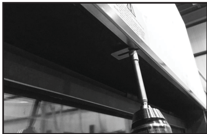
Figure 10.5. Install Trim Ring
