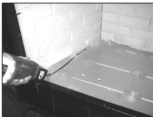
Figure 10.3. Using a saws-all, cut out the floor.
