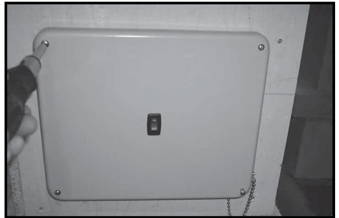
Figure 5.9 Replace Control Cover
