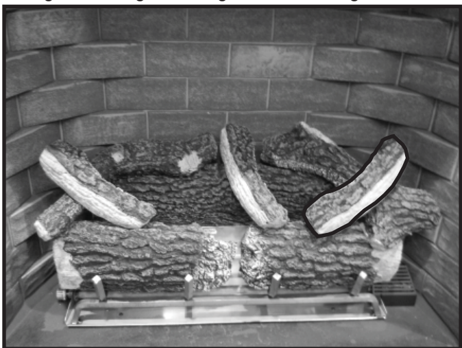
Figure 8.13 Place Right Center Log
