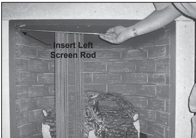
Figure 8.16 Insert Screen Rod
