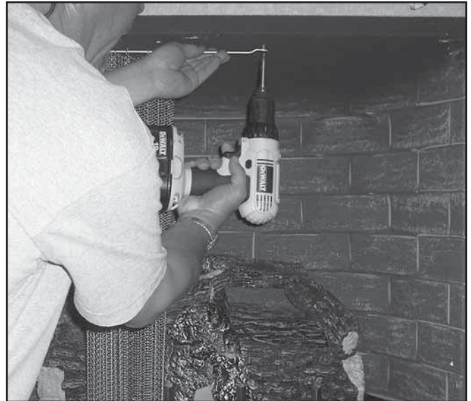
Figure 8.17 Fasten Screen Rod to Firebox Top
