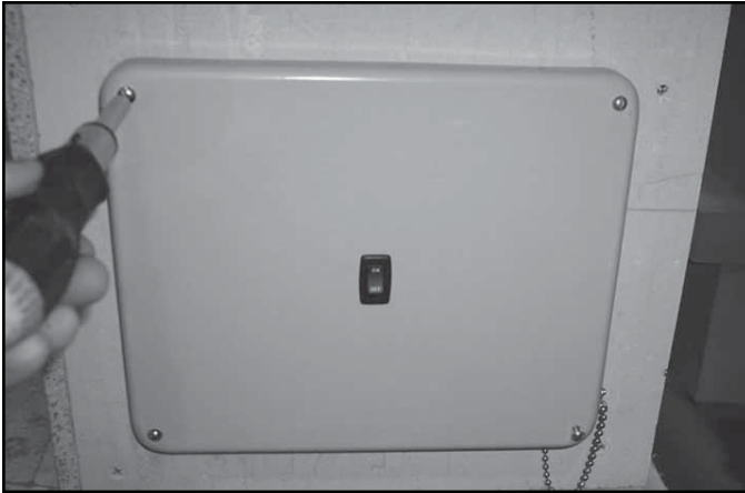
Figure 5.1 Remove Control Cover
