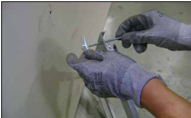
Figure 4.5 Toggle Bolt Installation through Mounting Bracket
