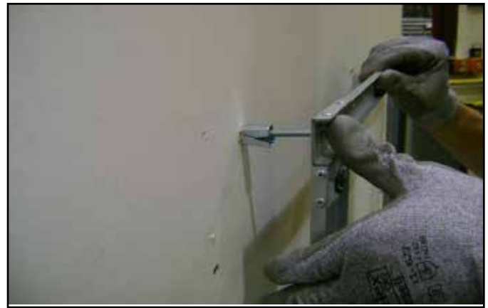
Figure 4.6 Installing Anchors in Hollow Wall
