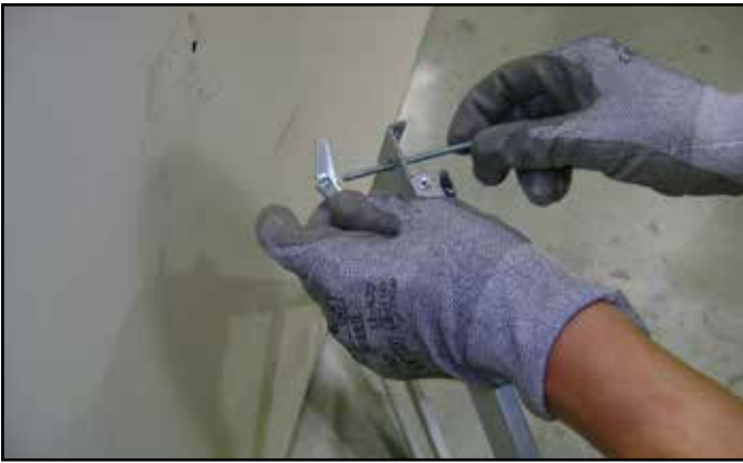
Figure 4.5 Toggle Bolt Installation through Mounting Bracket
