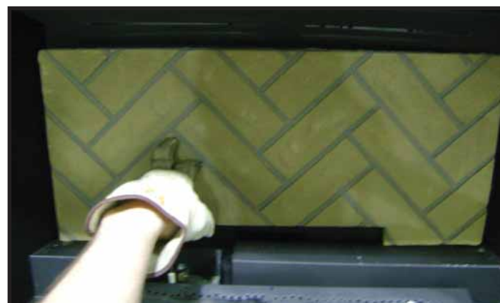
Figure 2. Install Back Refractory
