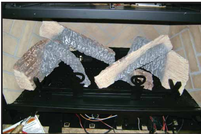
Figure 2. Refractory and Logs Installed
