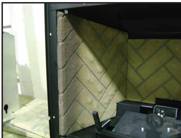
Figure 3. Install Side Refractory
