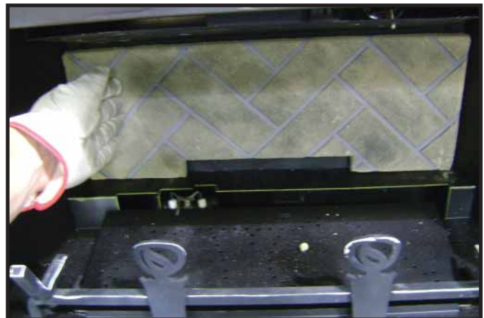
Figure 3. Install Back Refractory
