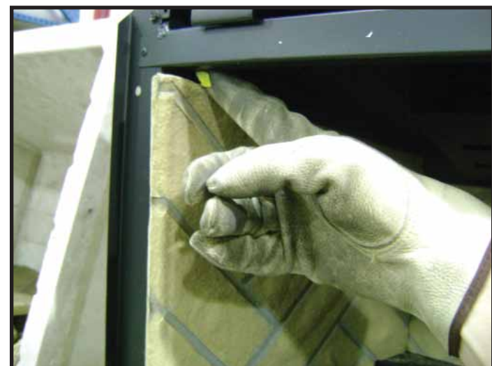
Figure 5. Bend Refractory Tab
