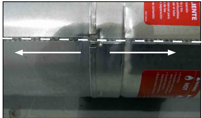
Figure 7.8 Align and Disassemble Vent Sections
