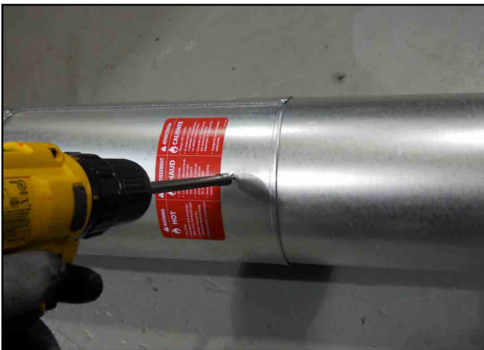
Figure 7.4 Screws into Slip Section
