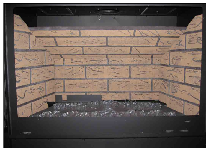
Figure 10.8 Refractory Installed
