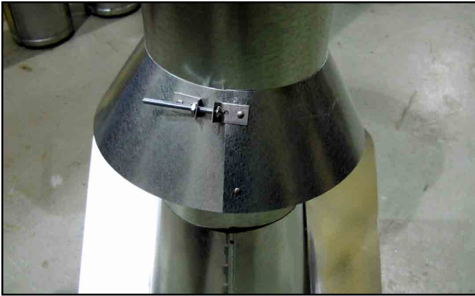
Figure 7.14 insert Bolt into Brackets
