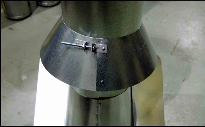
Figure 7.14 insert Bolt into Brackets
