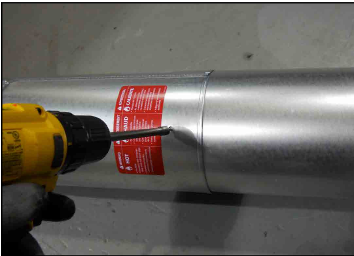
Figure 7.4 Screws into Slip Section
