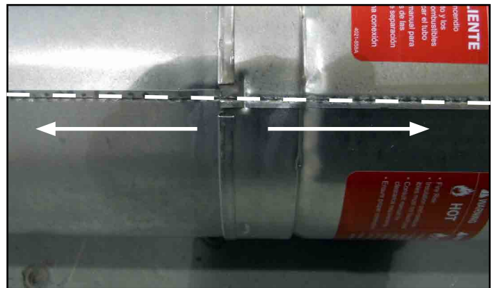
Figure 7.8 Align and Disassemble Vent Sections
