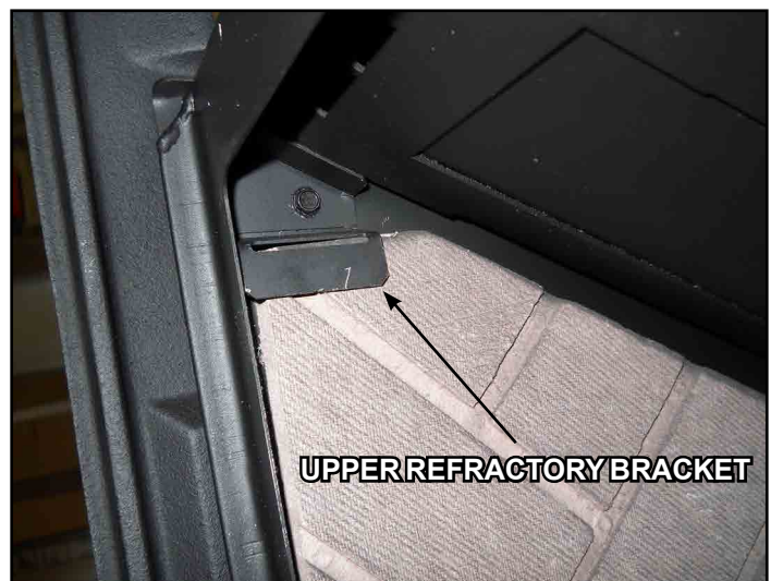
Figure 10.7 Upper Refractory Brackets
