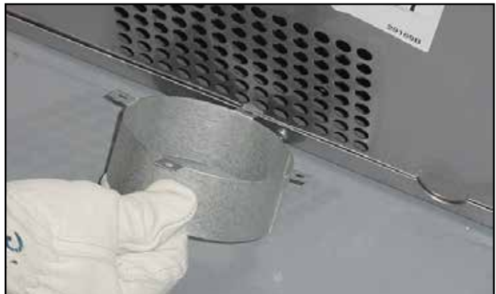
Figure 4.1 Slide the Tabs
