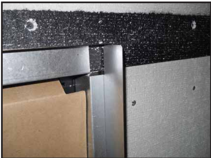
Figure 10.5 Finishing Template Bends
