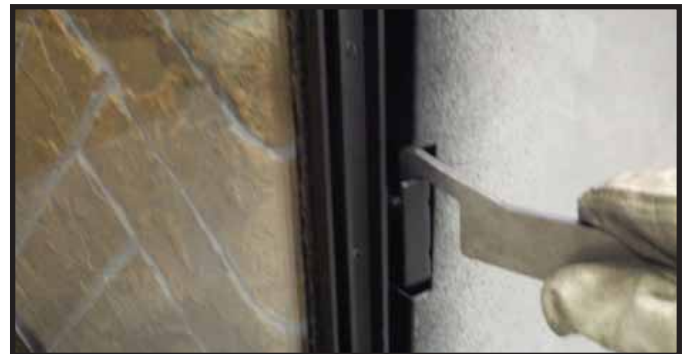
Figure 11.7. Securing Side Glass Clips
