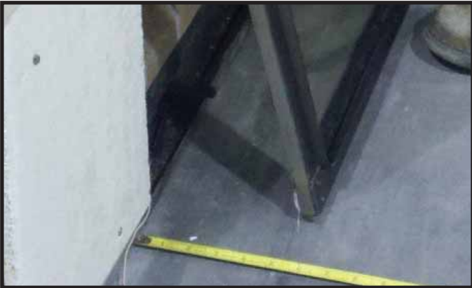
Figure 11.4 Positioning Glass
