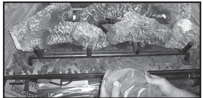
Figure 14.3 Placement of Lava Rock
