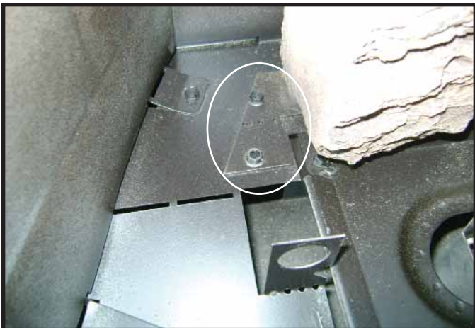
Figure 3.4 Remove Screws from Log Tabs
