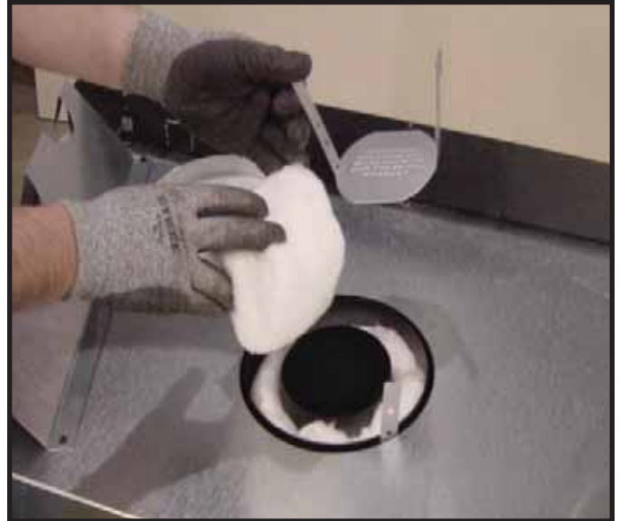
Figure 9.4 Remove the insulation basket and white insulation from the center vent pipe.
