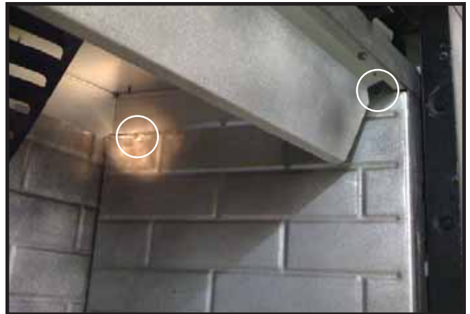
Figure 3.6 Top Screws For Metal Refractory
