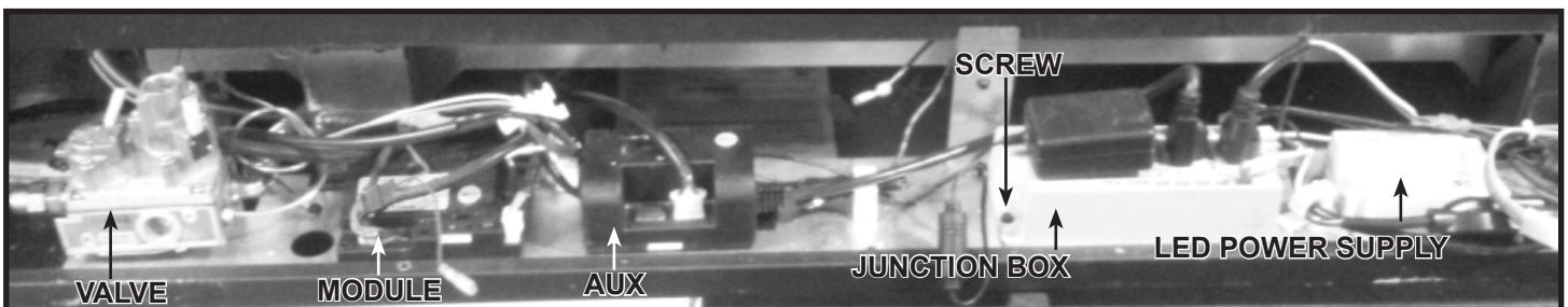
Figure 8.4. Valve Cavity (Lower Access Cover Panel Removed)
