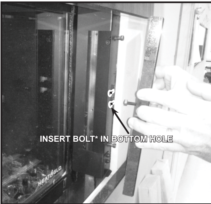
Figure 10.25. Install Side Granite Pieces
